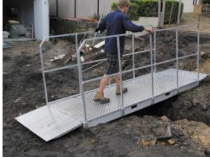
a) Prefabricated bridge (Sinclair 2017)
