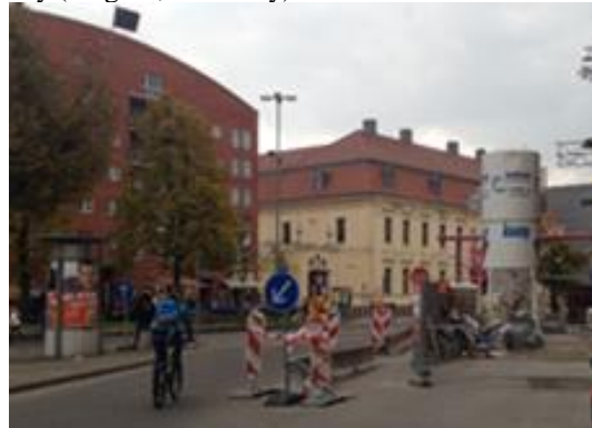
c) Cyclist share the lanes while pedestrians are provided a protected temporary walkway (Berlin , Germany)
