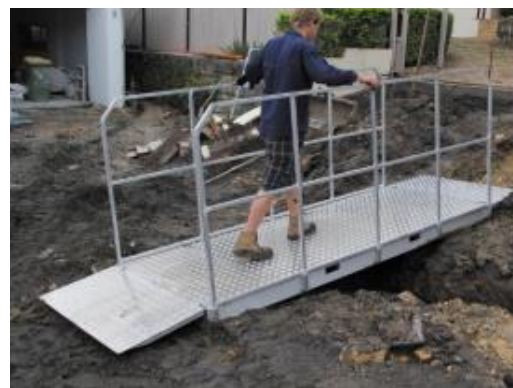
b) Use of a temporary prefabricated bridge
