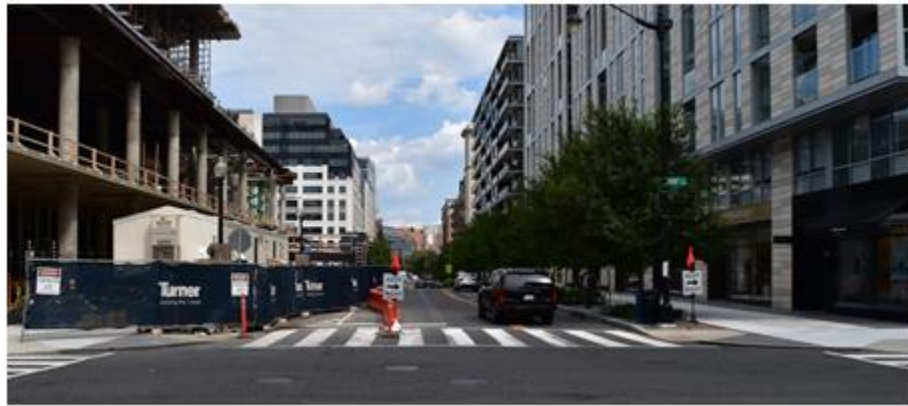
Figure 2-15. Non-motorized traffic is detoured via the nearest sidewalk
