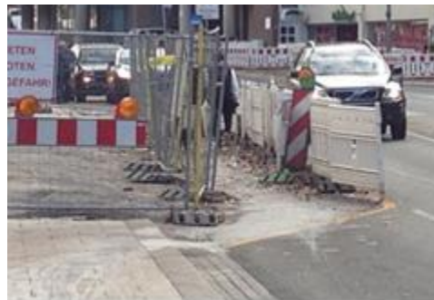
c) A close up view of the walkway surface condition
