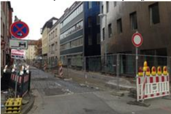
e) Part-width construction
