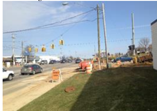
c) Closed sidewalk on South Westnedge Avenue (Picture 2)
