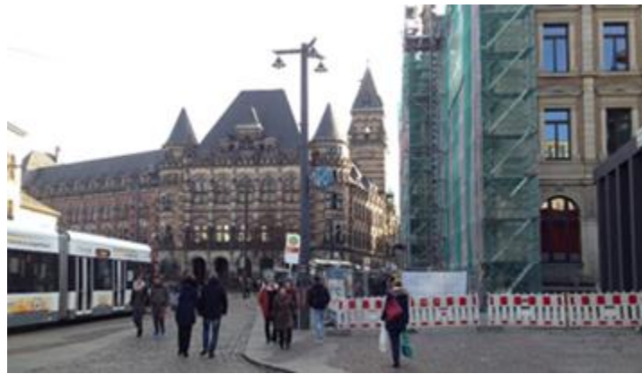
a) A work zone designated for a building renovation project
