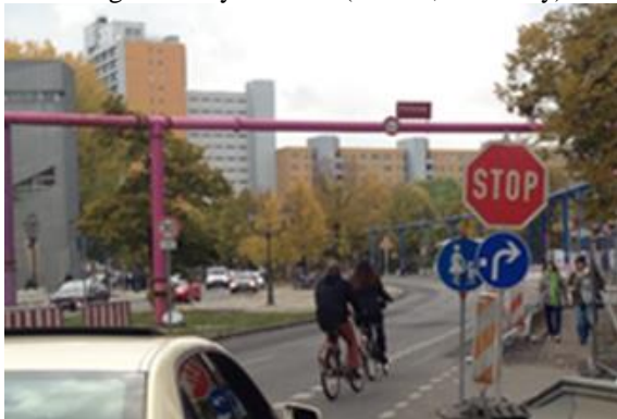
d) A temporary bicycle lane and a protected walkway (Berlin , Germany)
