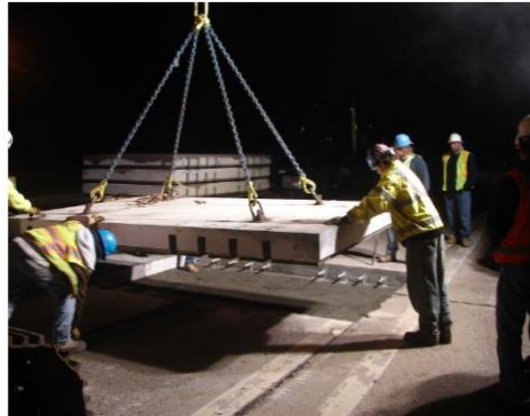
Figure 2-27. Precast concrete slab being lowered into place (Snyder 2012)
