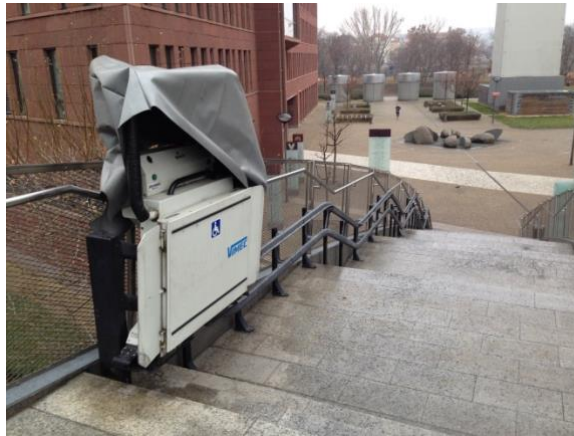
b) Platform of trolley system
