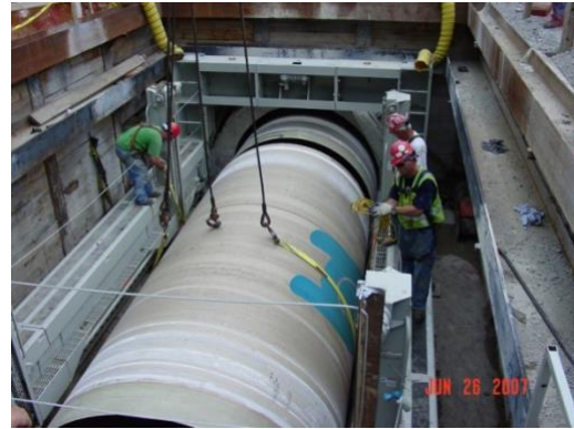
b) Segmental sliplining (HOBAS Pipe 2017)
