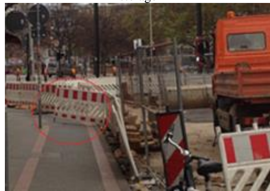
d) Improper management of fences/barriers
