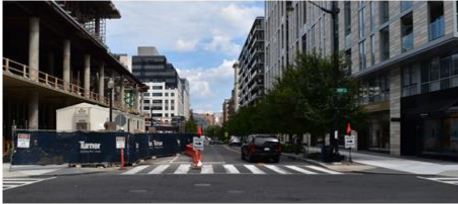
Figure 4-11. Non-motorized traffic is detoured via the nearest sidewalk (Washington DC)
