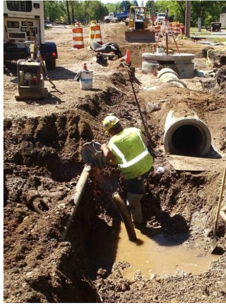
a) Traditional open-cut pipe replacement
