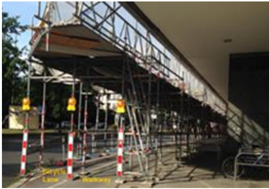
a) Covered bicycle lane and walkway (Steglitz, Germany)
