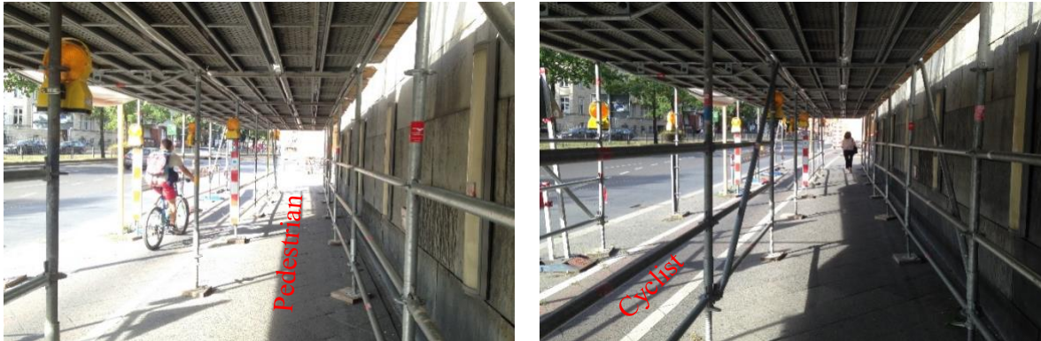
Figure 2-9. Separate access for pedestrian and cyclist
