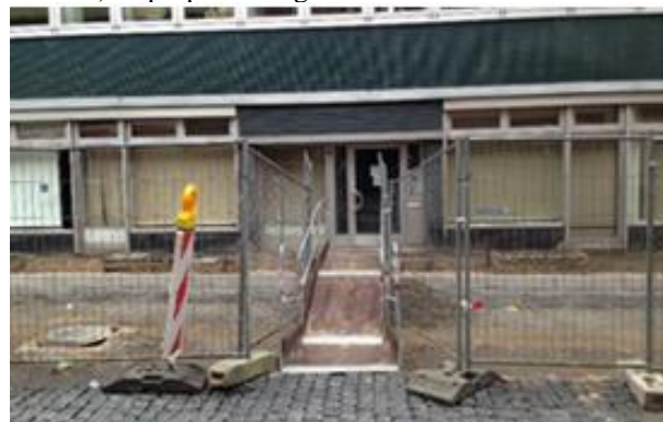
f) Use of a temporary bridge
