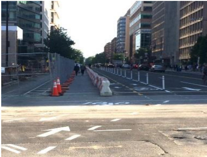
a) Separated pedestrian and cyclist temporary pathway
