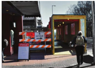
b) Covered way made of wood for pedestrians (Raleighnc 2017)
