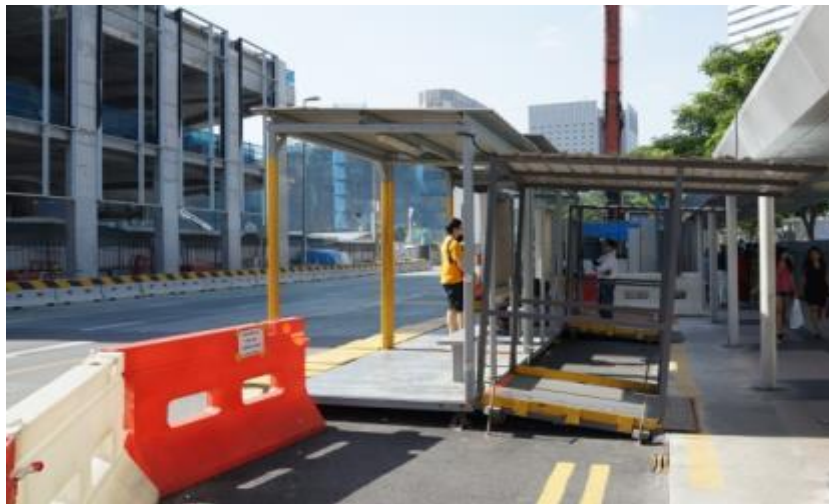
a) Relocated transit facility with a temporary shelter
