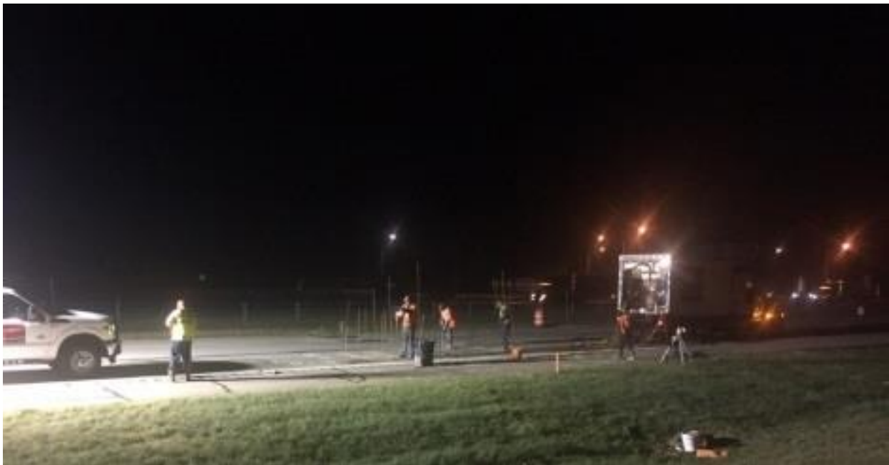
b) Nighttime slab jacking, slab stabilization, and soil densification
