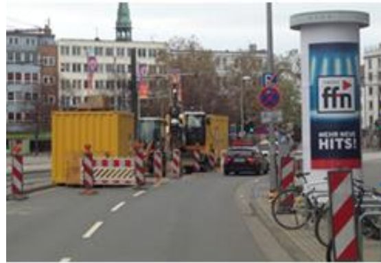
b) A lane occupied for construction activities and storage
