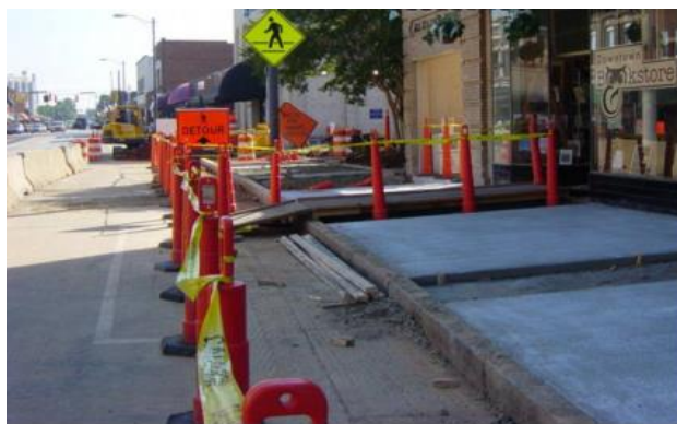
a) Phase construction was performed to provide access to shop
