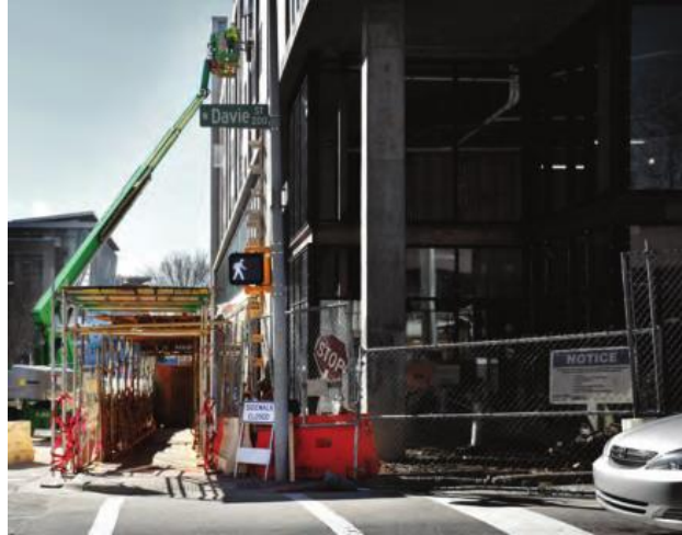
Figure 2-7. Covered walkway (Raleighnc 2017)
