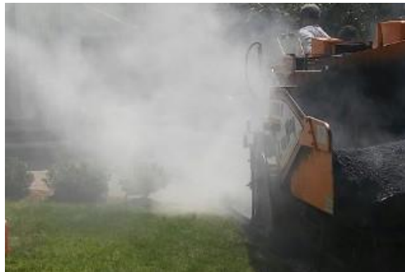
b) Hot mix asphalt (HMA) paving (Eddy's Construction 2016)
