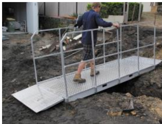
Figure 4-10. Prefabricated bridge (Sinclair 2017)
