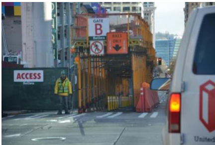
a) Covered way made of scaffolding for bicyclist (Sinclair 2017)
