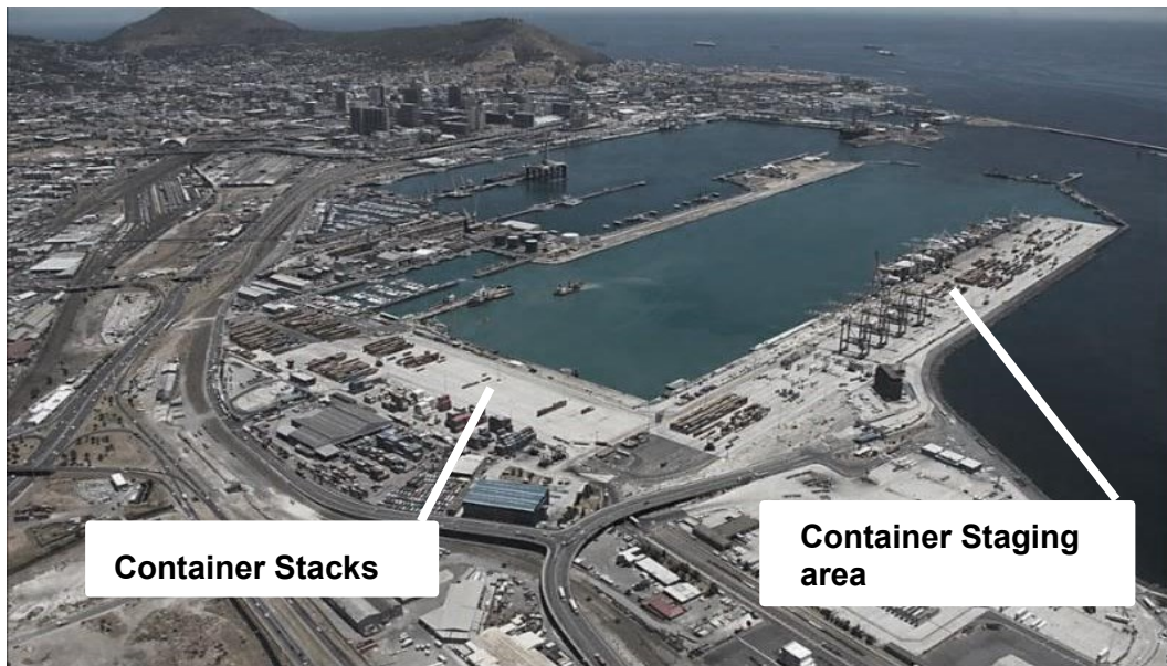
Figure 5-18: Aerial photograph of the Cape Town Container Terminal
