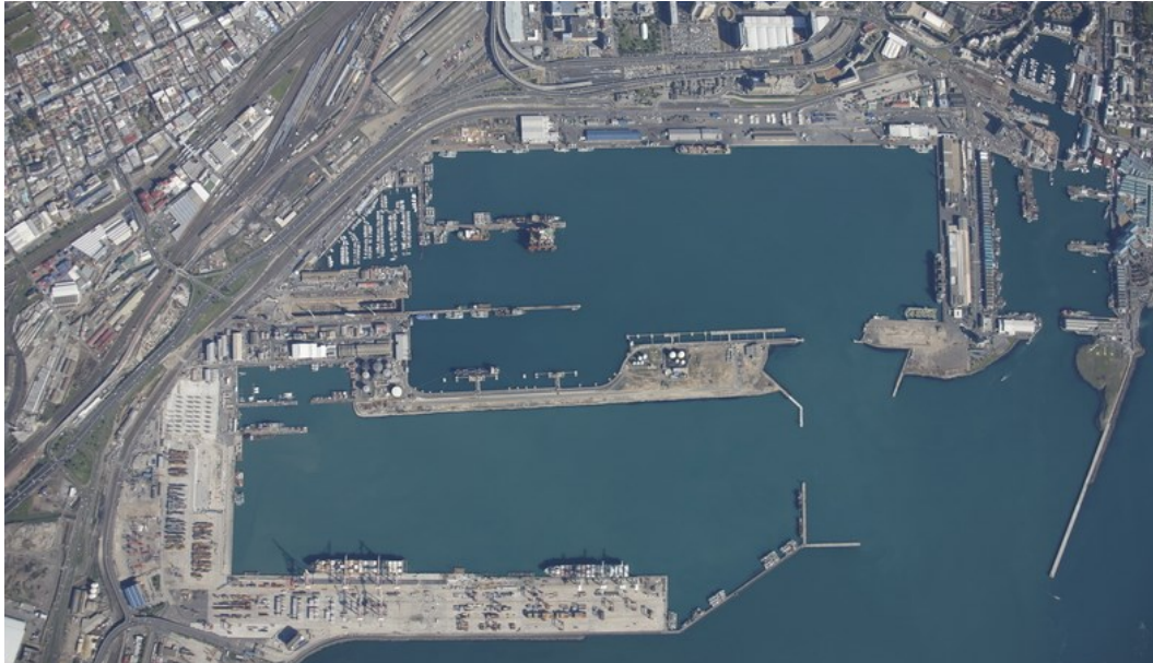
Figure 5-10: Aerial Photograph of the Port of Cape Town
