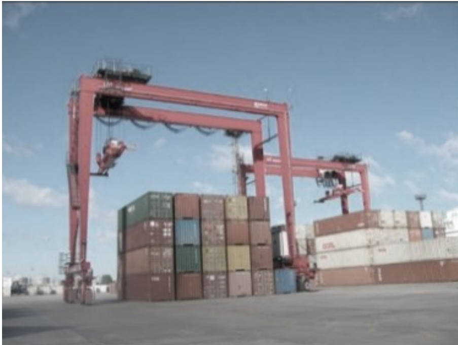
Figure 5-21: Rubber Tyred Gantry Cranes, CTCT
