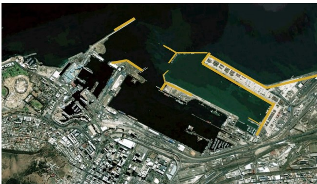
Figure 5-8: Construction of the Ben Schoeman Container Terminal in 1975
