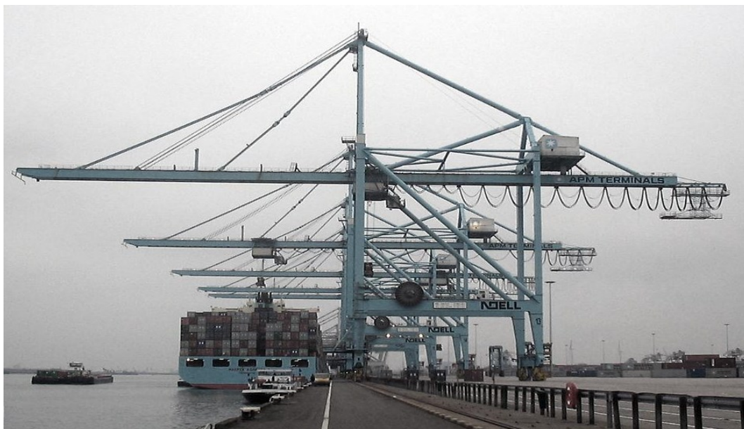
Figure 5-20: Super-post-Panamax cranes similar to those in the CTCT
