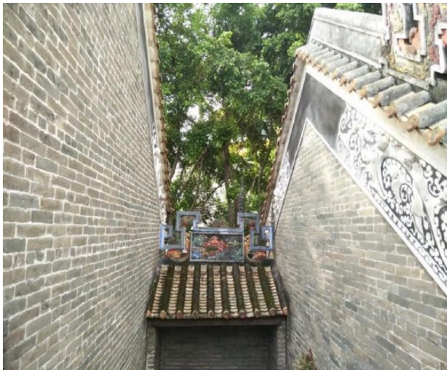
Figure 3. Restoration of stone painting and carvings.
