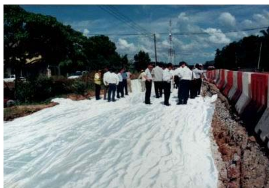
Figure 2: The use of geotextile to improve soil condition
