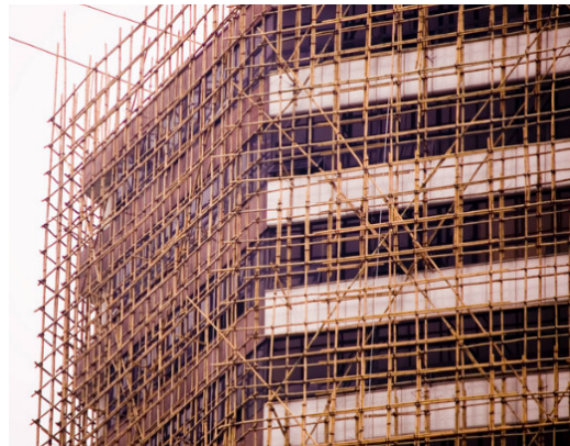
(b) Bamboo Scaffolding [6]
