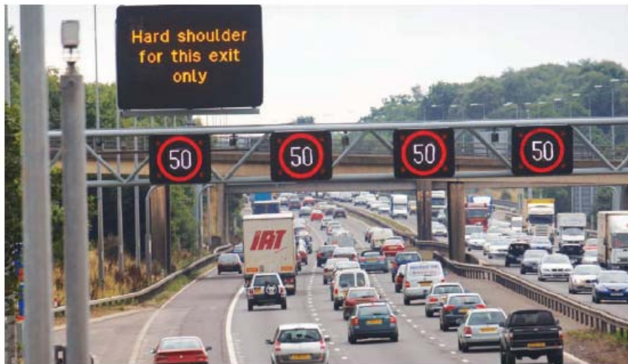
Figure 1.3: Use of Intelligent Transport Systems on the M42 in England [4]
