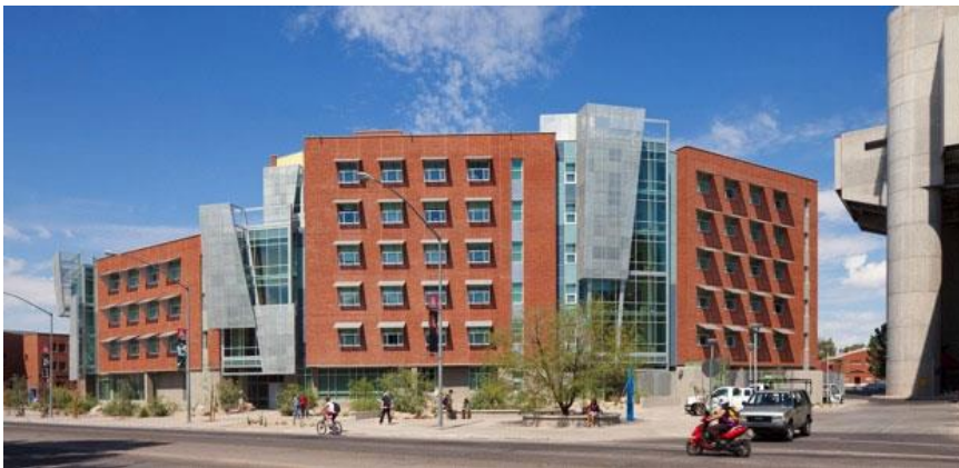
Figure 1 Likins Hall Building
