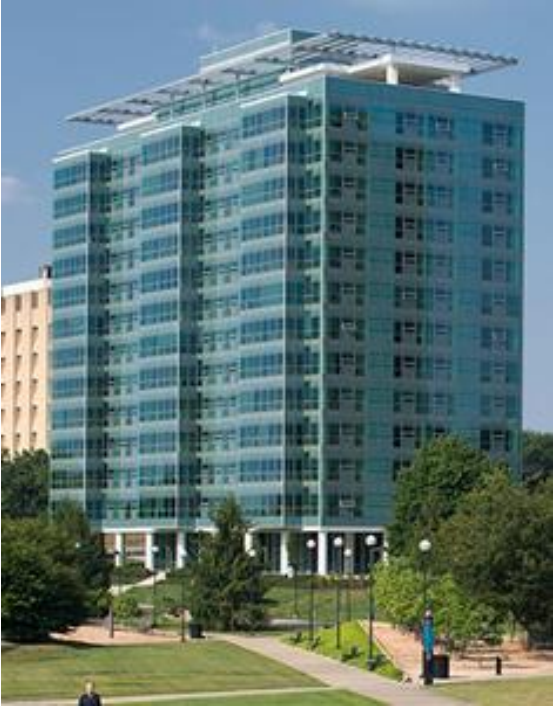
Figure 28: The Exterior of Mogens Hall
