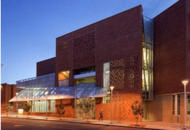
Figure 2: The Likins Hall Main Lobby
