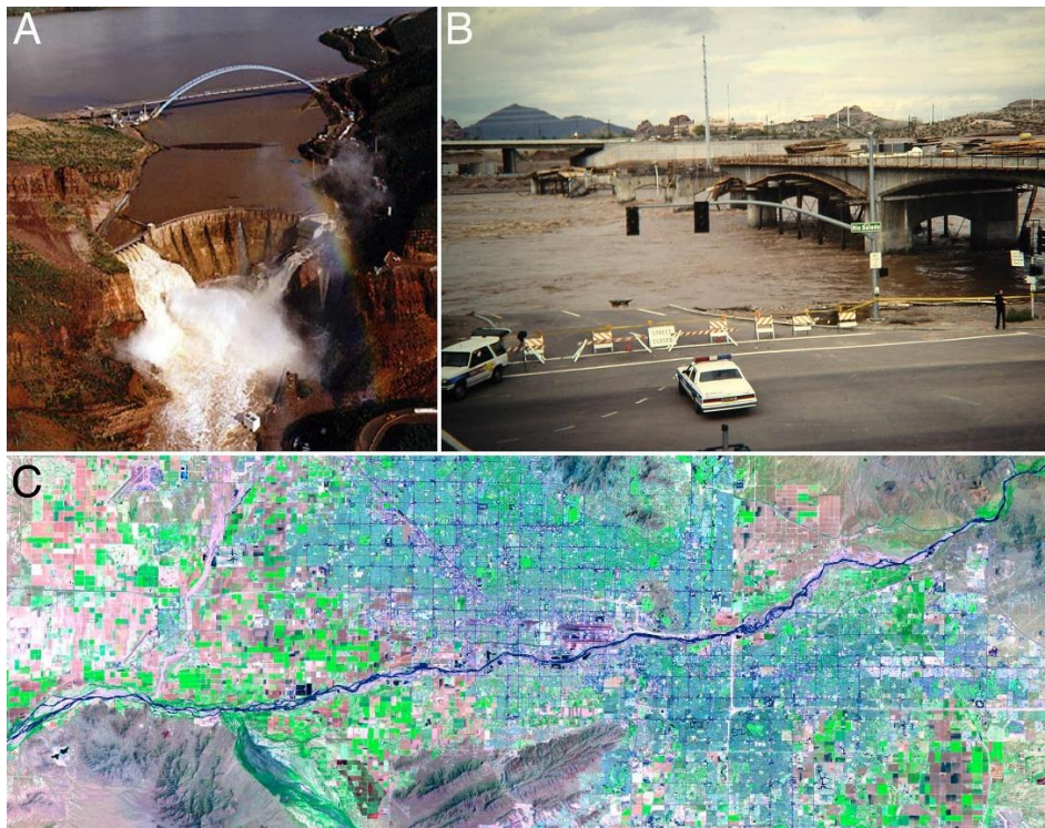
Figure 2.20. During the winter of 1993, a major ENSO event led to (A) the release of water from the reservoir behind the Roosevelt Dam. The released water destroyed the bridge at Mill Avenue in Tempe (B), as well as other infrastructure along the course of the river through metropolitan Phoenix (C).
