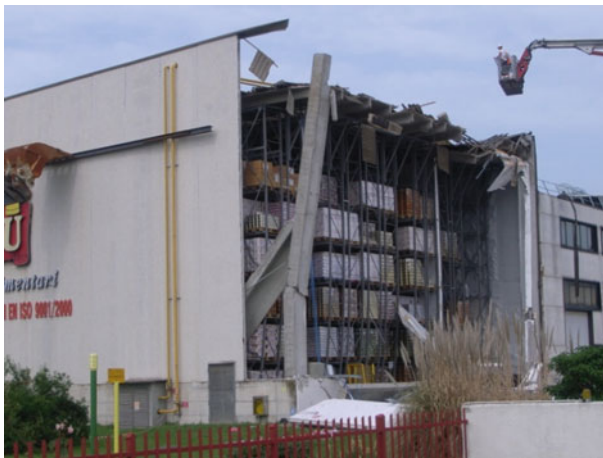
Fig. 11 Partial collapse of the roof, longitudinal girders, column and front cladding of a flat roofed precast building
