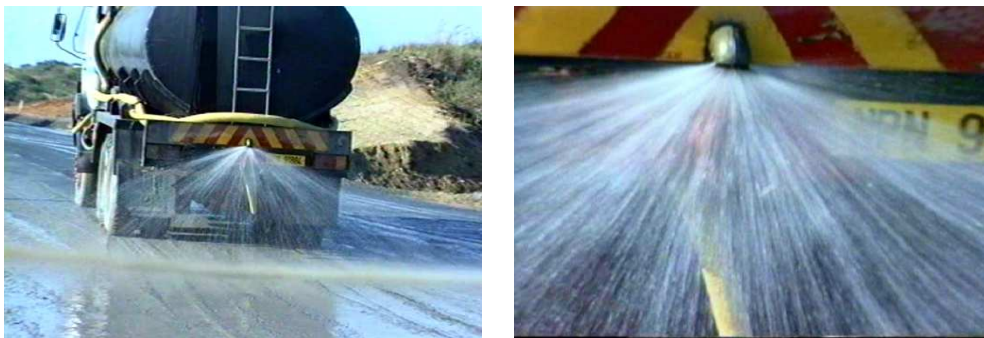
Figure 17 The tank truck at the begging of Slushing Process
