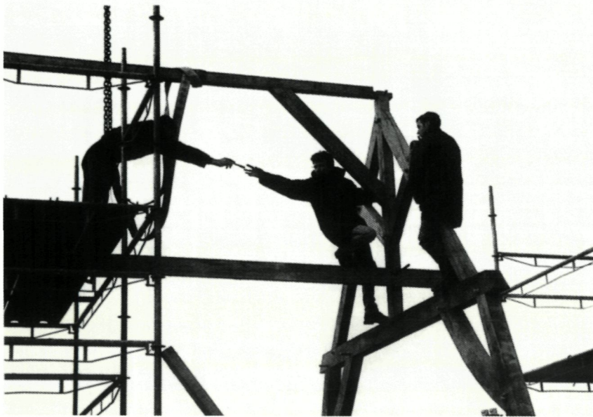
8 A carpenter reaches for a timber pin to secure a roof timber.
