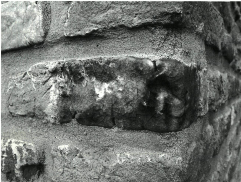
4 A mediaeval brick with unusually extensive natural glazing, re-used in the wall of a reconstructed house.
