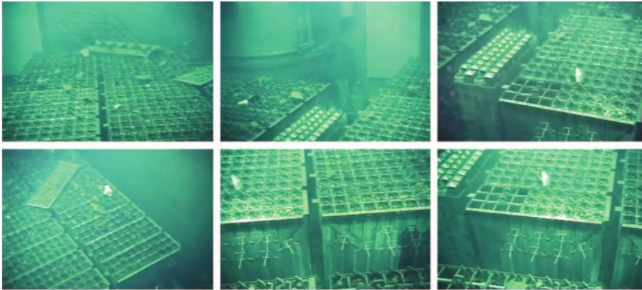
Figure 1.9: Photographs of the above-reactor spent fuel storage pond in Unit 4 obtained using a remotely-operated underwater vehicle by TEPCO. From [59].
