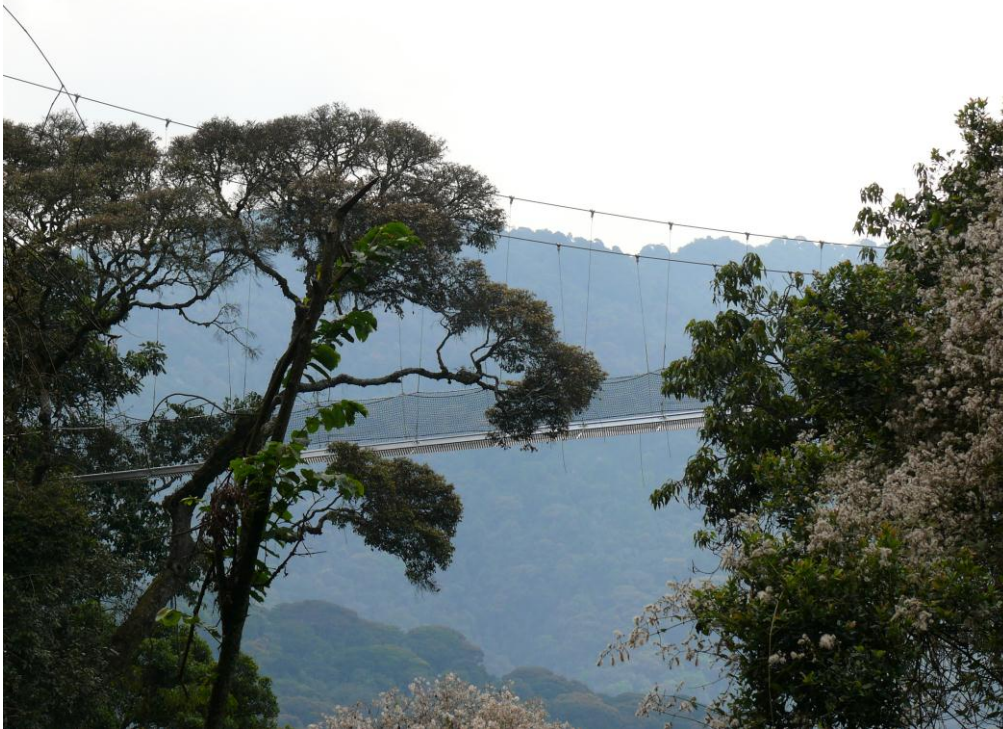
Picture 3: The Nyungwe canopy walkway in Rwanda was built by Greenheart Conservation Company Ltd. in 2010. The construction consists of three towers, three platforms and 165m of bridge connections.
