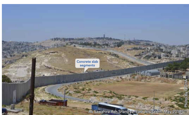
(a) Concrete barrier
