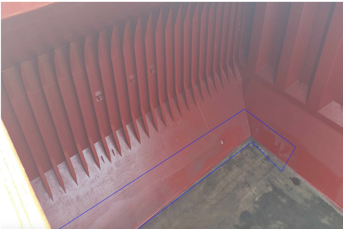
Figure 45 - Completed application of Epoxy N top coating on board No.4 (P) Cargo Hold of Post Panamax Bulker - Case A. Blue line denotes application area.
