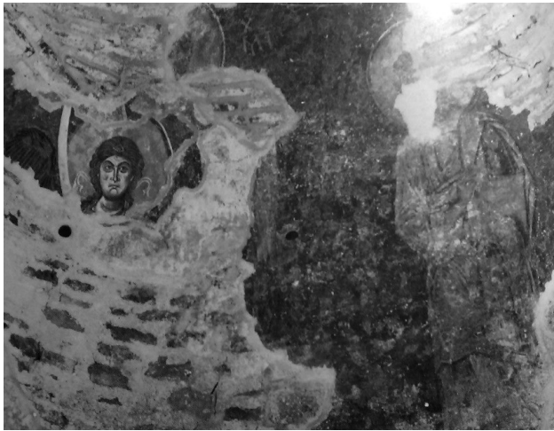
Openings of acoustic vessels in the Church of Sts Peter and Paul in Novi Pazar (Source: Нешковић & Николић 1987)
