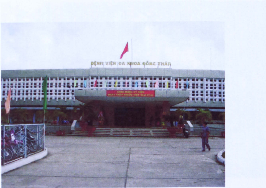
Figure 2.3 Dong Thap General Hospital in Cao Lanh City at the Mekong Delta, Southern Viet Nam. (Photo by Mai Ngọc Lanh)
