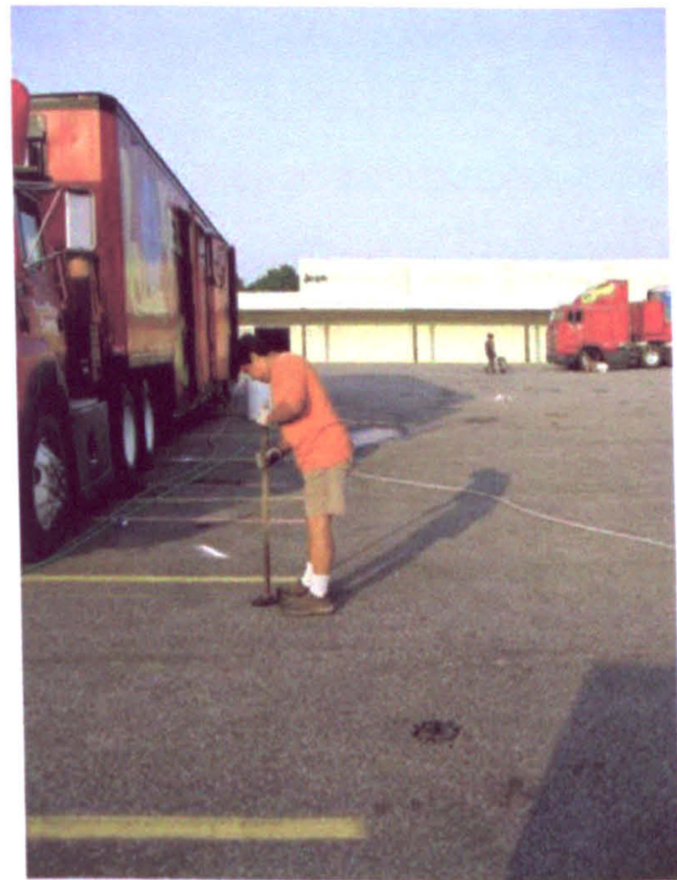
Figure 3.16: Filling holes in Greenville, PA on July 27.
