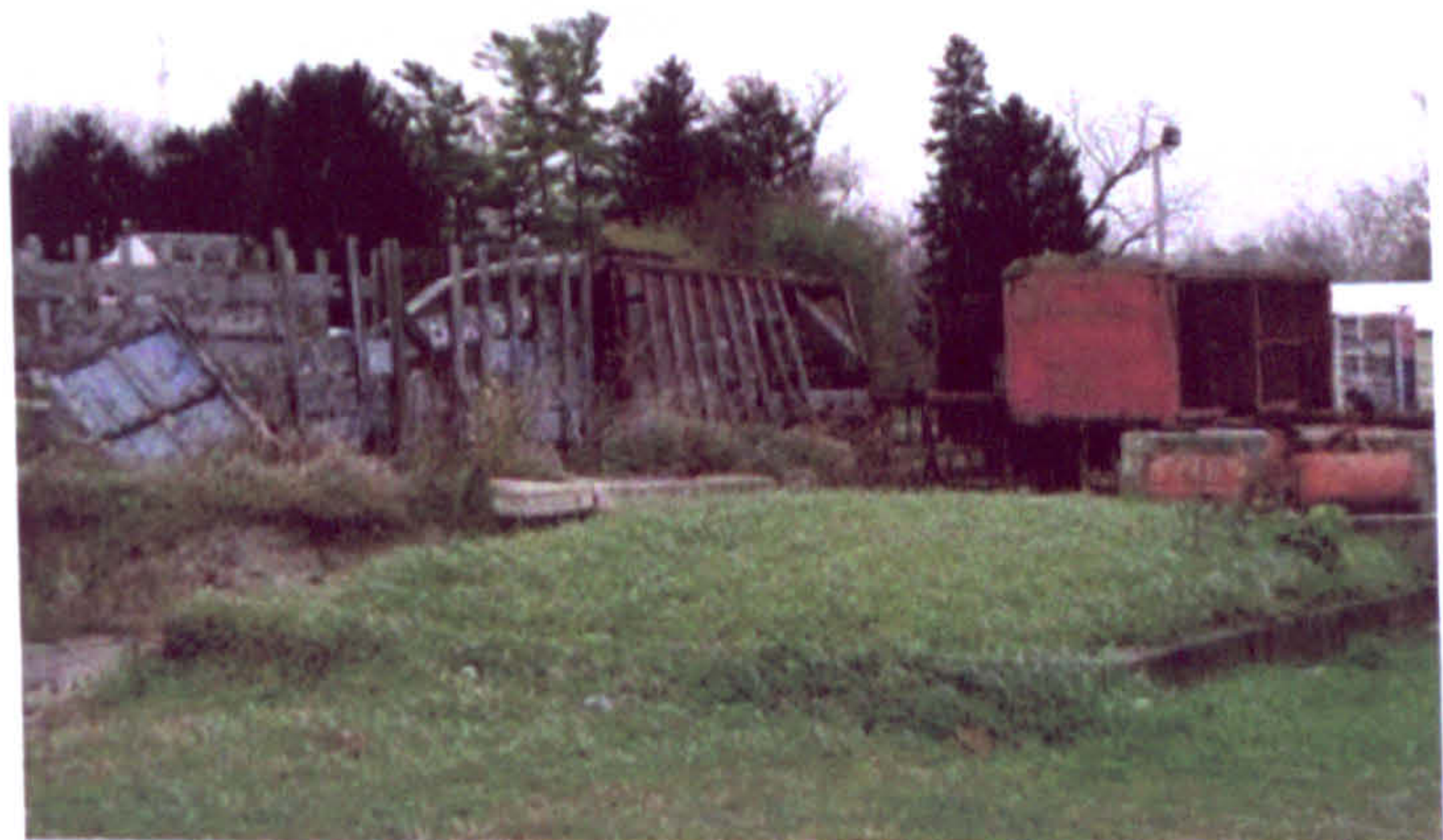
Figure 2.17: The International Circus Hall of Fame in Peru, IN on November 15, 2007. Circus wagons slowly giving themselves to the soil as they wait to be restored.
