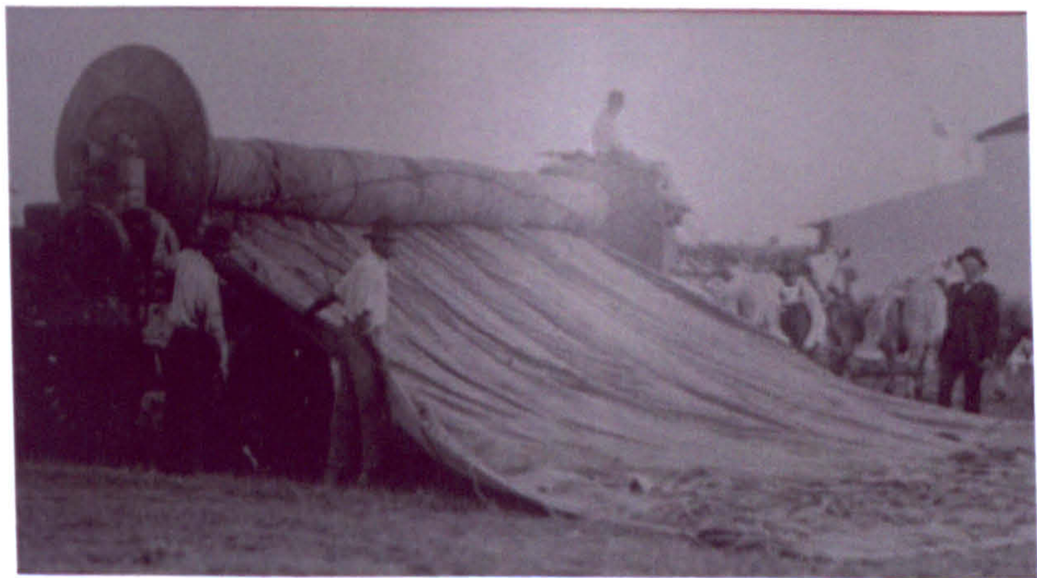
Figure 3.11: An early version of a tent spool truck. Photo taken at Circus World Museum.
