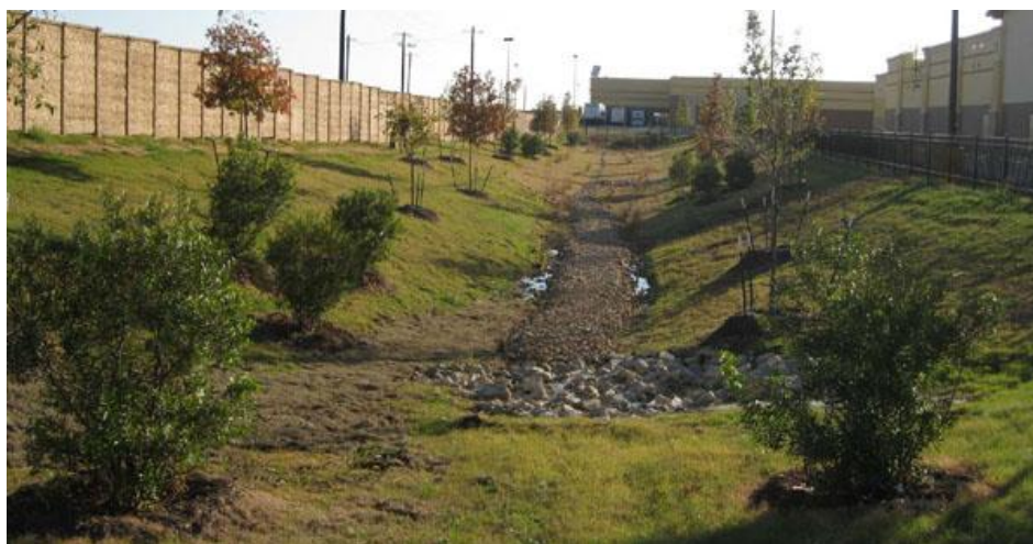
Figure 42. Bioretention at Rayzor Ranch, Denton, Texas. (Retrieved from http://iswm.nctcog.org/Documents/iTools/Case_Studies/Rayzor_CS.asp )
