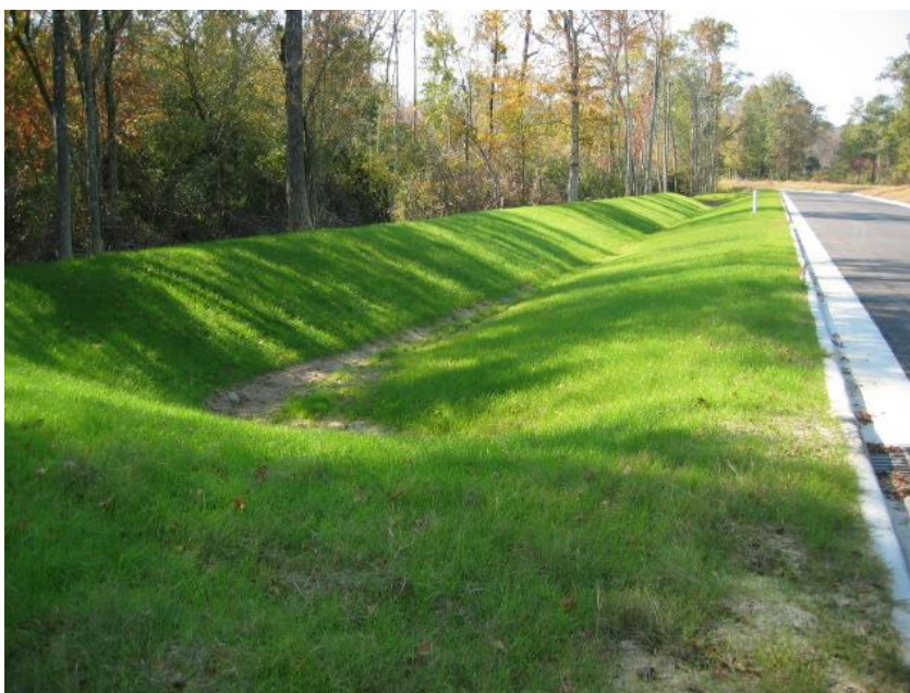
Figure 34. Grass swale example at Sellhorn Heights in New Bern, NC (Retrieved from http://www.thomasengineeringpa.com/photo_gallery/photo_gallery.htm ).
