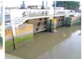
Crest gate to regulate water levels upstream. © P. Baran
