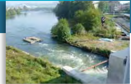
View of the complete eel-recovery system with the VLH in operation. © Ecogea
