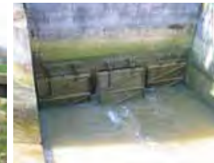
Flaps to regulate water flow. © P. Baran
