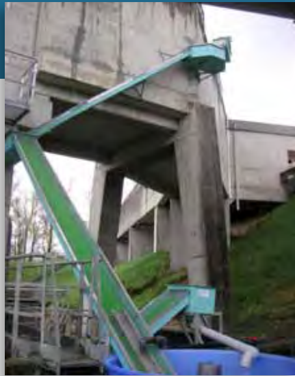
Brush pass with ramps and rest basins at the Golfech dam. © L. Carry
