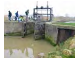
Tide gates and flaps opened during ebb tide. © P. Baran
