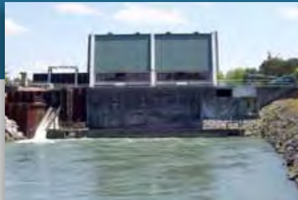
Hydroelectric plant seen from downstream. © P. Gomes
