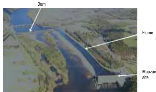
Aerial view of the Mauzac plant (© EDF).
