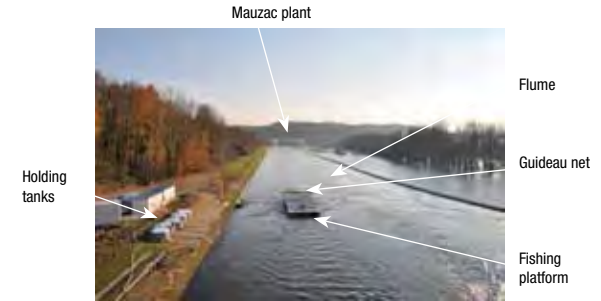
The flume upstream of the plant (© ECOGEA).
