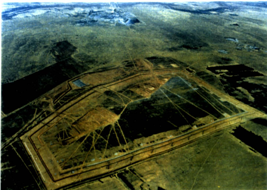
Figure 4: Aerial photograph of the construction phase of Mispah slimes dam.
