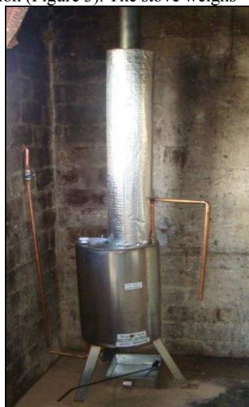
Figure 3. Photograph of the Shiza Manzi biofuel geysers in a farm house
