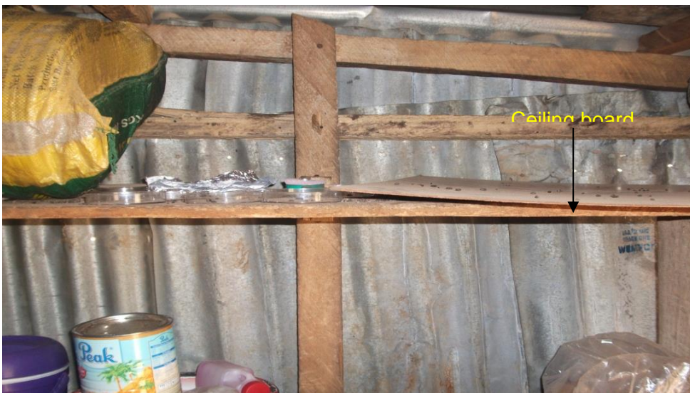
Plate A-2 Collection of settled dust on a ceiling board placed on a shelf in a local kitchen
