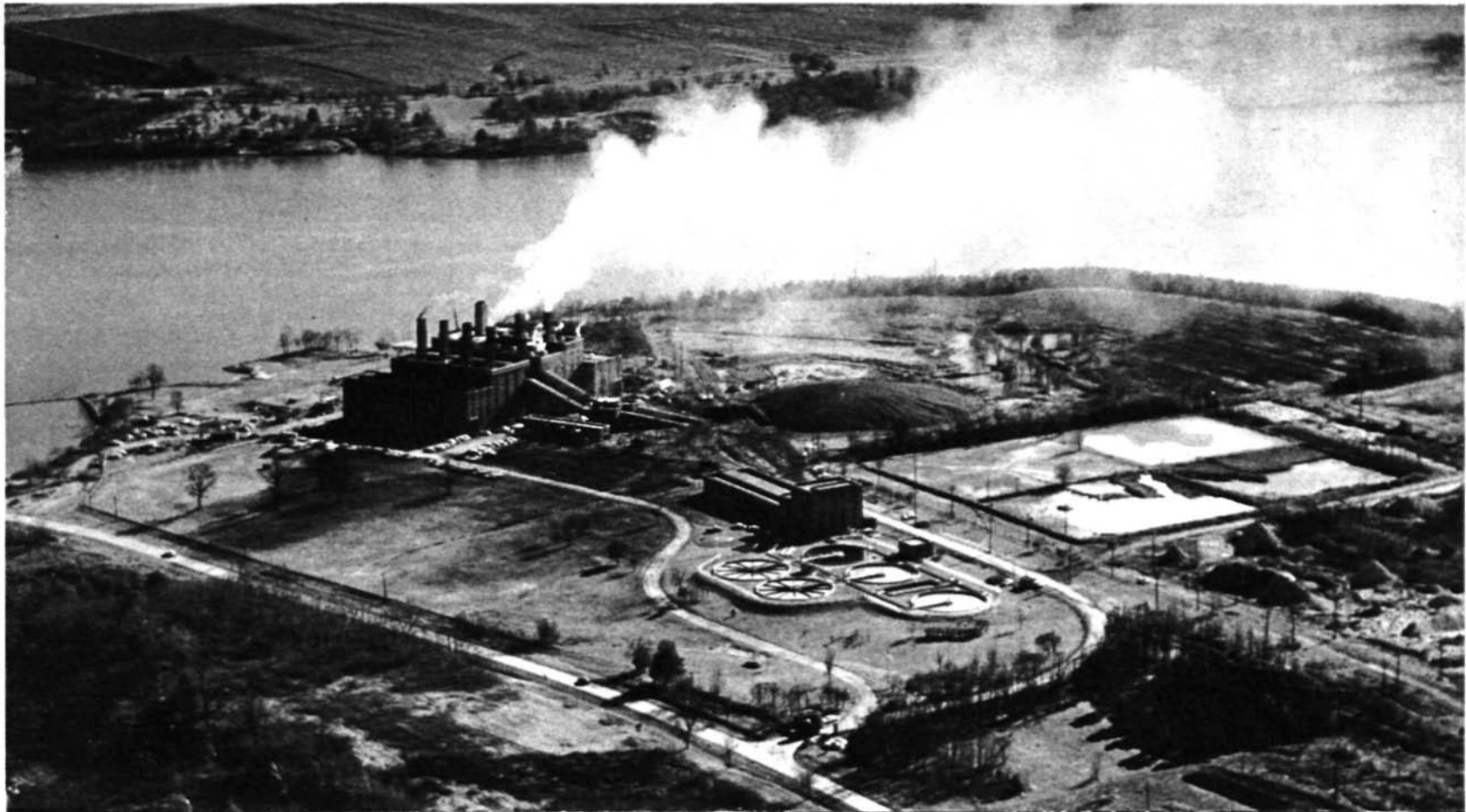
Water treatment plant at Springfield
