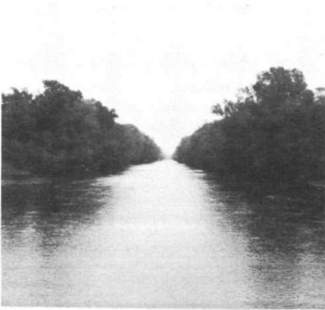
FIGURE 2 Looking east into Indiana (upstream) from the State Line Bridge, we see the straightened channel of the Kankakee River.
