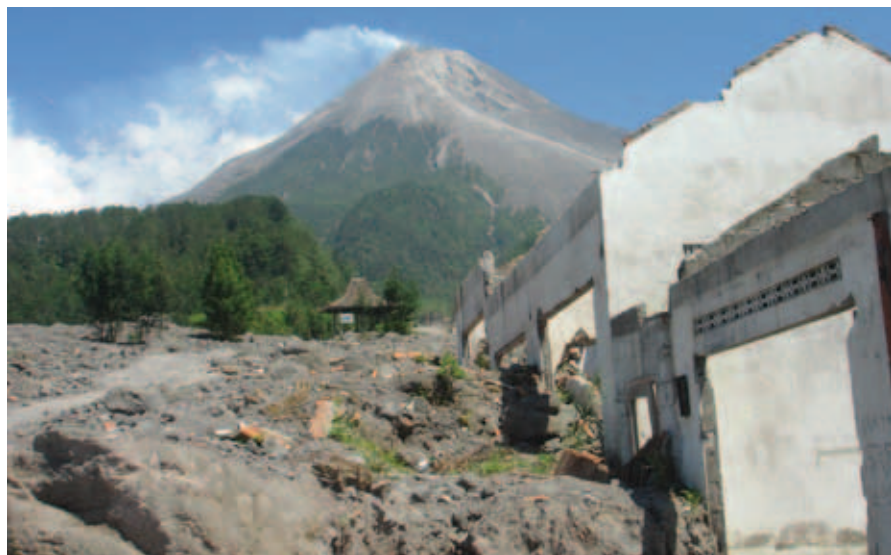
Extensive damage caused by the volcanic eruption of Mt. Merapi, Indonesia
