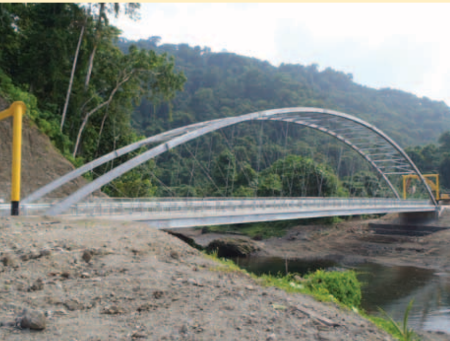
New high-level bridge in the village of Maepua. Makira, Solomon Islands
