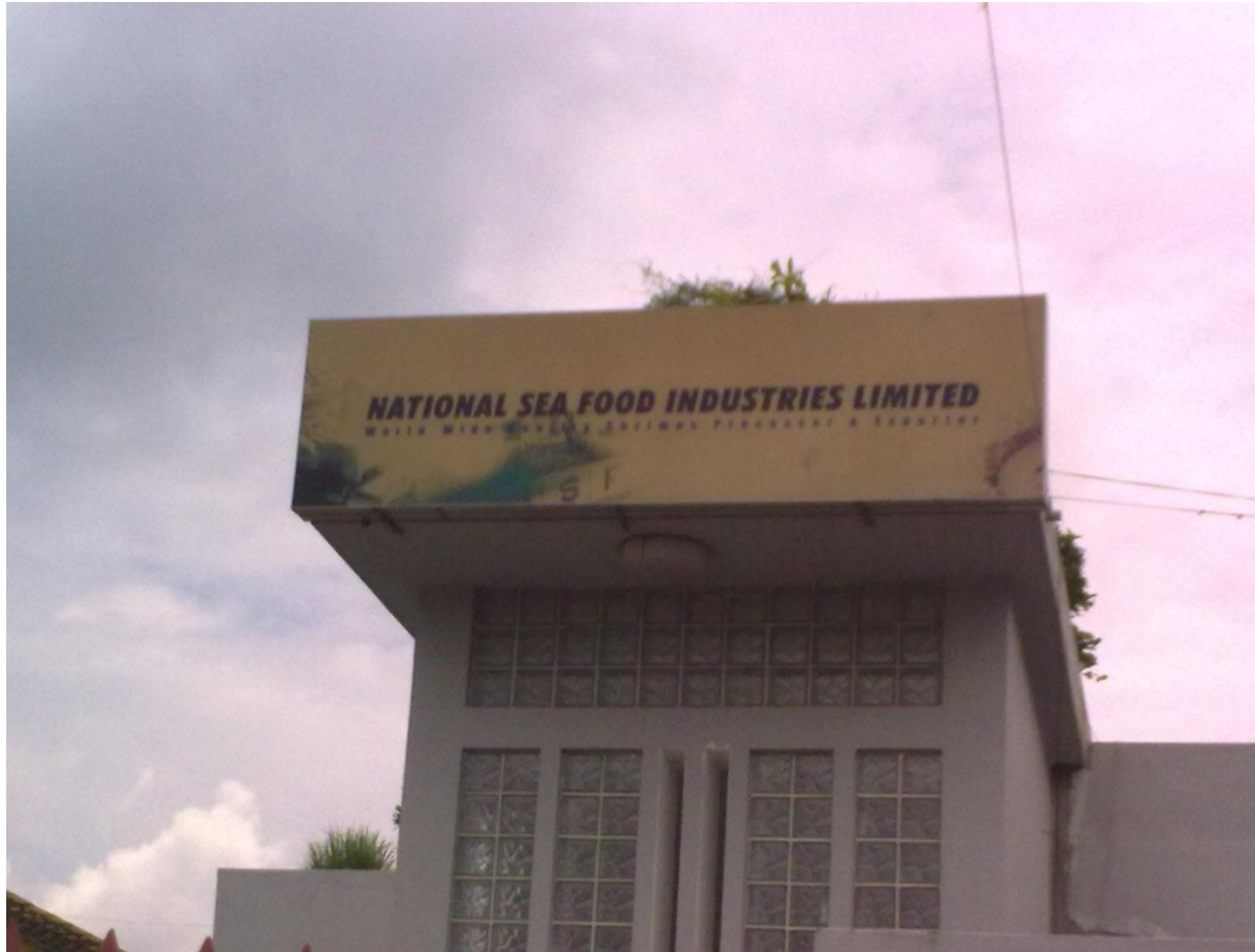
Figure 4 - Processing plant - Verite photo
