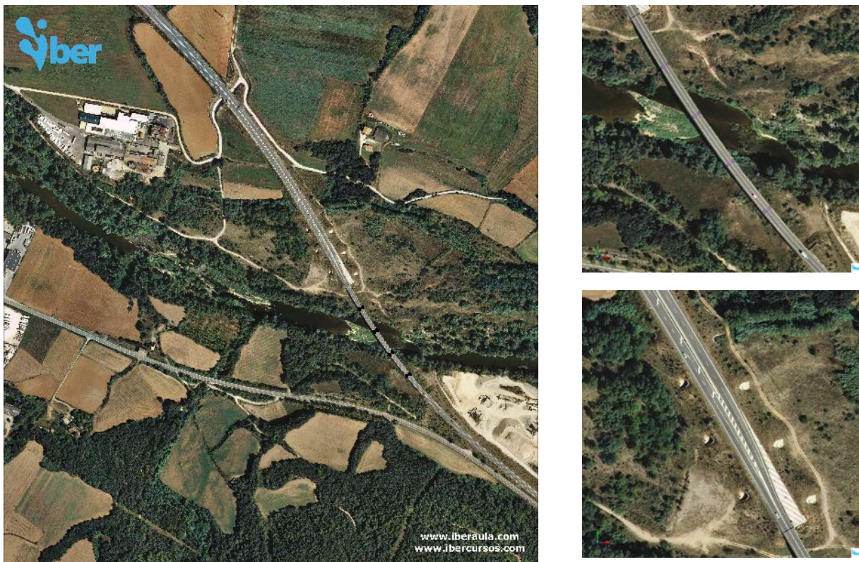
Figure 48. Study area. View of the background image (left), the geometrical discretization of the piers (top-right) and the culverts (bottom-right).
