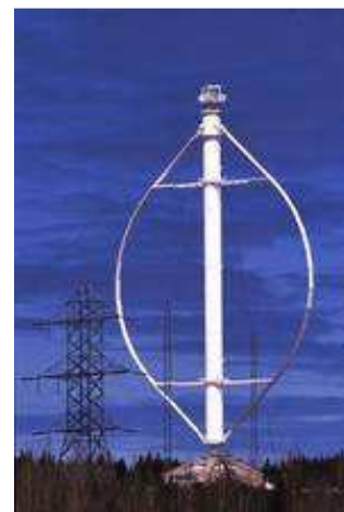
Fig. 13. Éole, the world largest Darrieus wind turbine.
