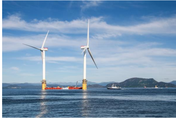
Figura 6: Parque eólico Hywind Scotland, Peterhead, Scotland [18]
