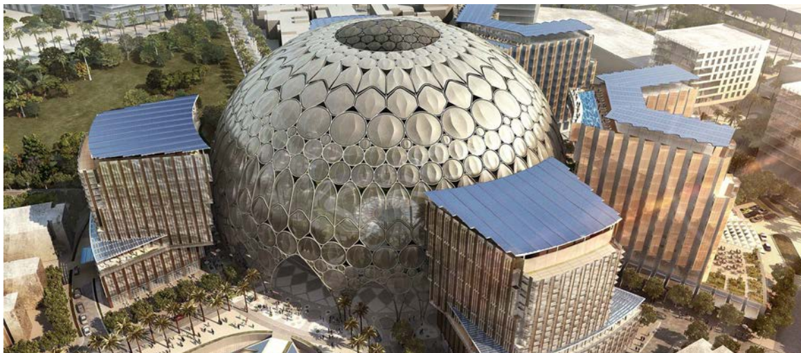
Figure 40: Al Wasl Plaza at Expo 2020 Dubai (Smith / Gill). New resources available for structural calculations have permitted the development of the innovative design of the interconnected rings of this gigantic 150-metre diameter metallic dome. (Source: AS+GG)
