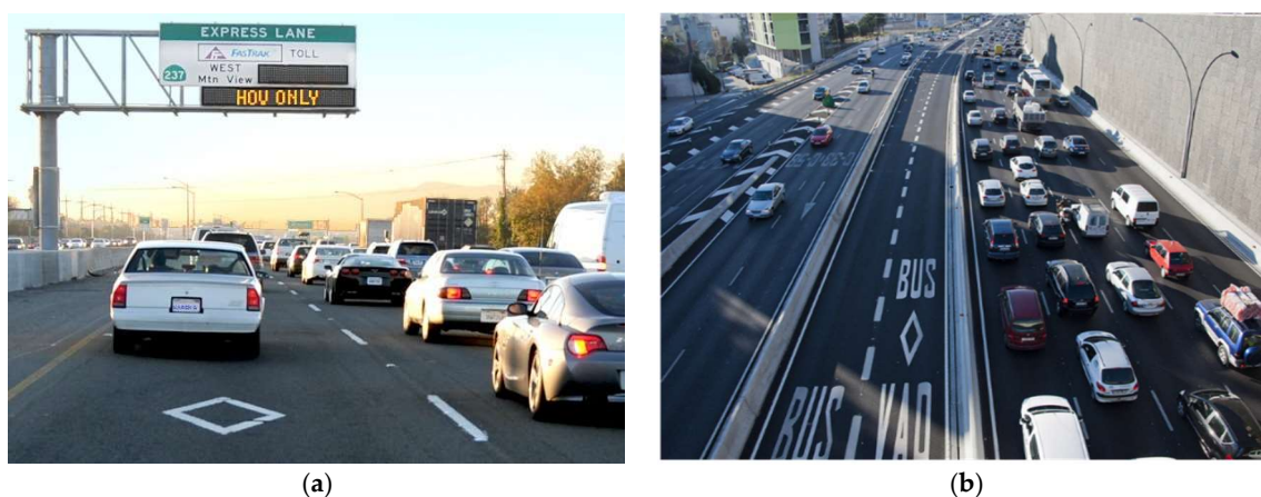
Figure 2. Dynamic versus static high-occupancy-vehicle (HOV) lanes: (a) adjacent HOV lane (Photo source: Nexobus); (b) segregated HOV lane (Photo source: Santa Clara Valley Transportation Authority, San Jose, CA, USA).
