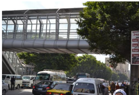
Fig. 7 the pedestrian bridge that in reality is not used by people.
