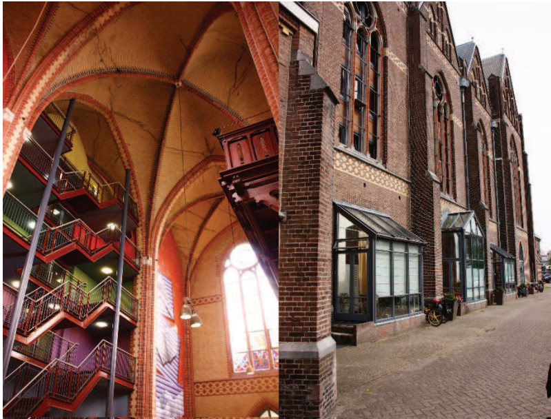
Fig.4: Two main consequences of a residential re-use can be found at examples like the Elbakerk in Haarlem (32). The addition of extra floors to create more ground space and also the addition of windows to ensure a sufficient lightning inside.
