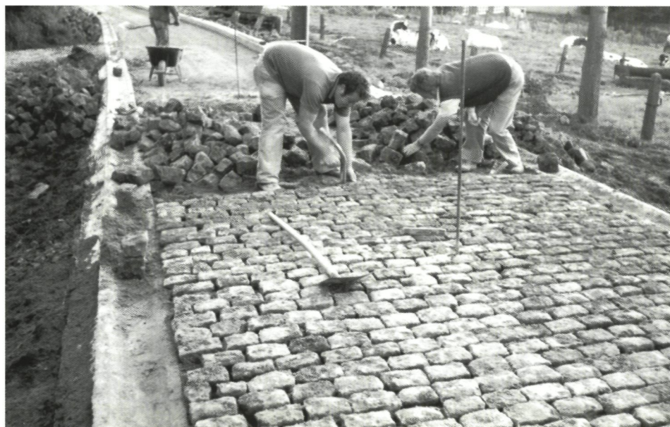
Figure 2. Paddestraat (Velzeke) during the works.
