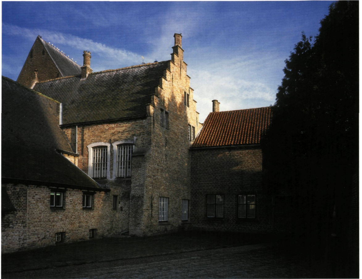
▶ 15th-century extension with stepped gable (photo K. Vandevorst)
