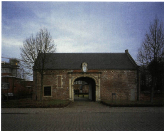
▶ Gatehouse from 1677 (photo K. Vandevorst)
