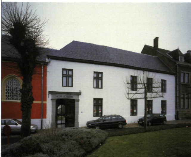
▼ Front of the hospital (photo K. Vandevorst)
