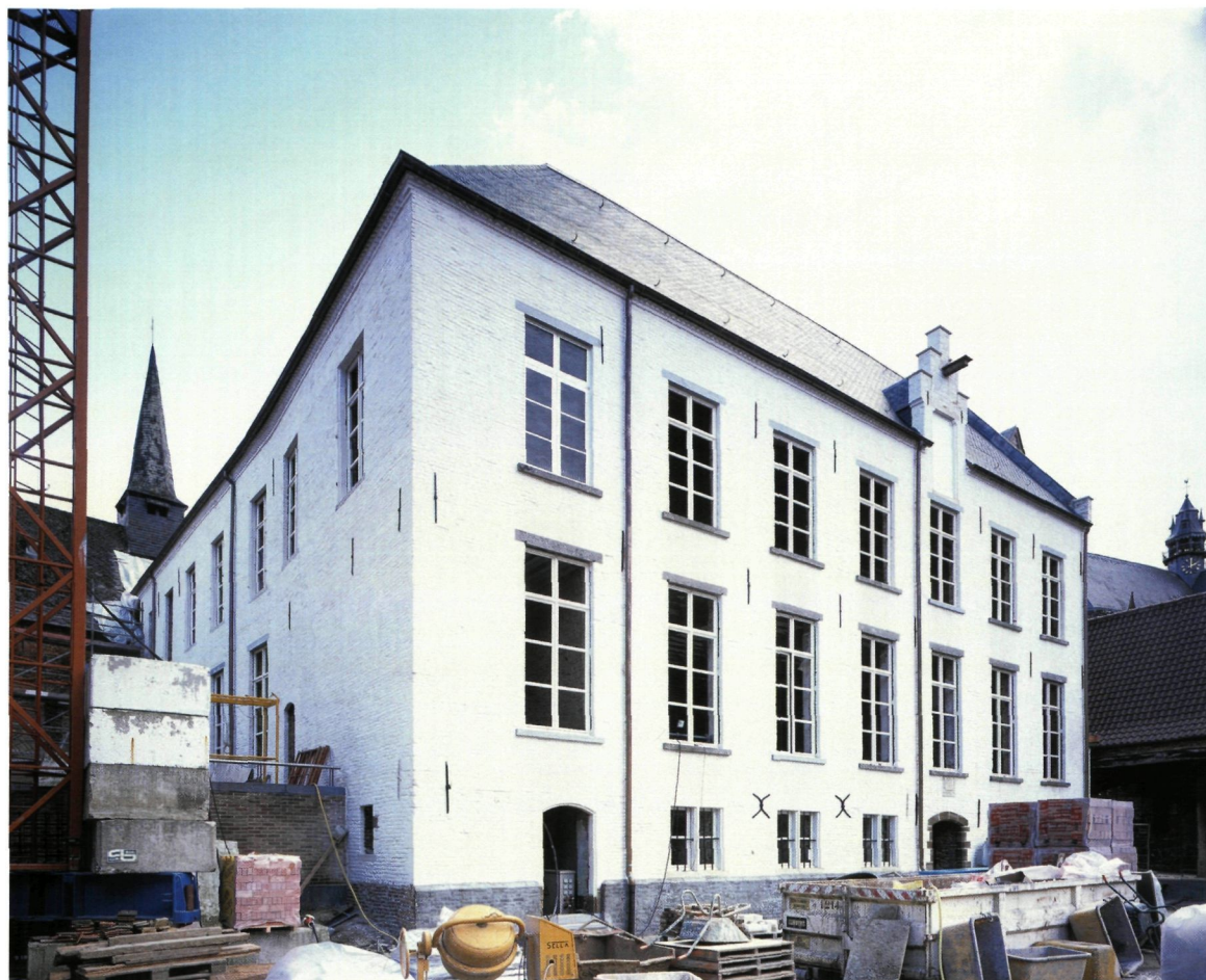
▲ Renovated part of the hospital (photo K. Vandevorst)
