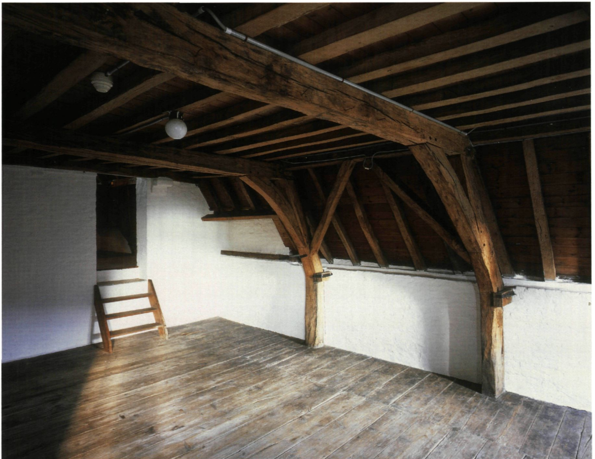
▶ Roof truss in the 15th century extension (photo K. Vandevorst)
