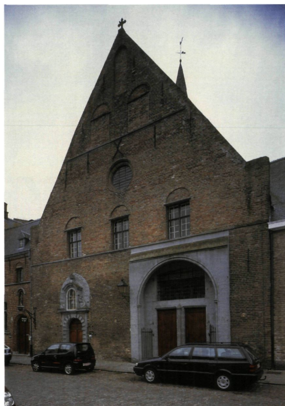
▼ Front of the hospital (photo K. Vandevorst)
