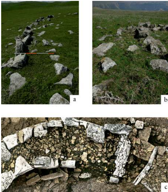
Fig. 7 Architecture details: double-framed walls. (a) Pravobereznaja Kičmalka 1; (b) Ransyrt 6; (c) Kabardinka 2, House 14. – Different scales.
