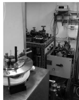
Fig. 2. Helium gas recovery system
