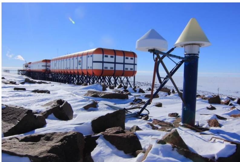
Figure 5: SANA E IV Ground Station
