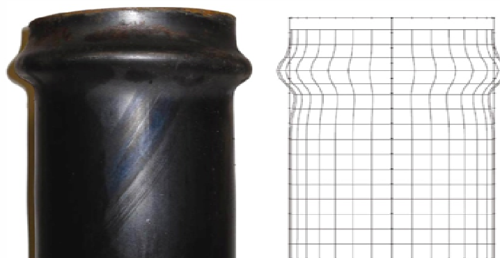
Fig. II.29 Failure mode known as “elephant foot”, typical in circular CFT sections. (Choi, 2007)
