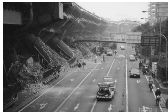
d) Shear failure of the Hanshin expressway, Kobe earthquake 1995
