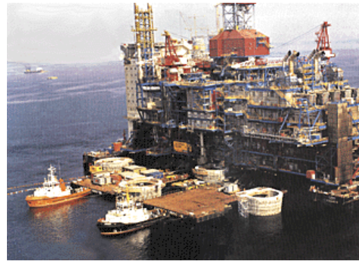
b) Sleipner offshore oil platform, Norway 1991
