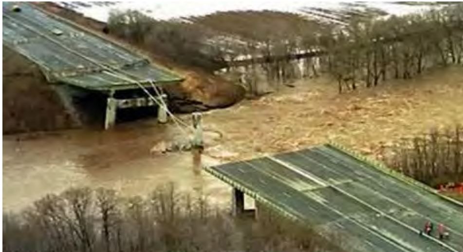
Figura 2. 7. Colapso del puente sobre Schoharie Creek. [Ref. www.bb.ustc.edu.cn ]
