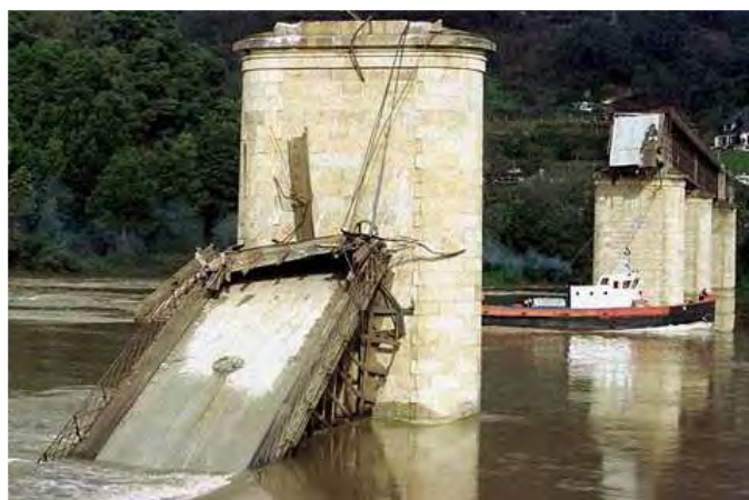
Figura 2. 8. Colapso del puente Hintze Ribeiro. [Ref. www.lumq.com ]
