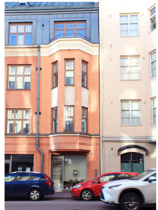
Image 8.2 Many old buildings in urban areas utilise bay windows to receive light from multiple directions and to open longer views along the street.
