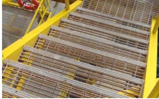
Figure 42 New gratings for staircase
