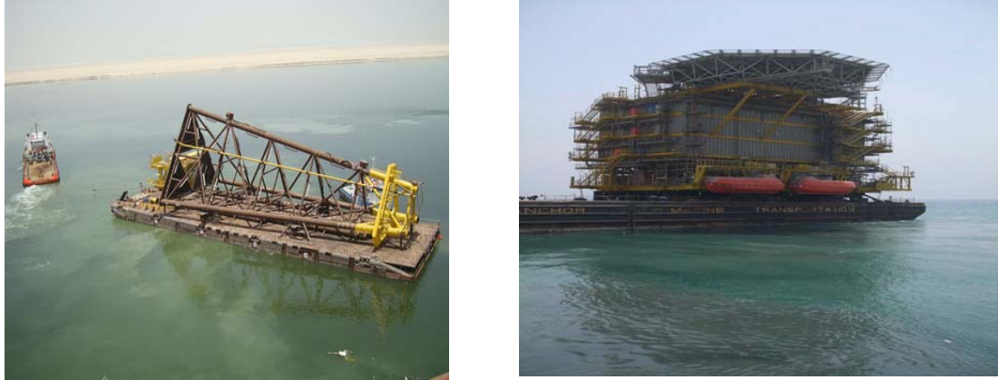
Figure 7 Jacket and topside sailing (Alyafei and Maerskoil Qatar, 2009)
