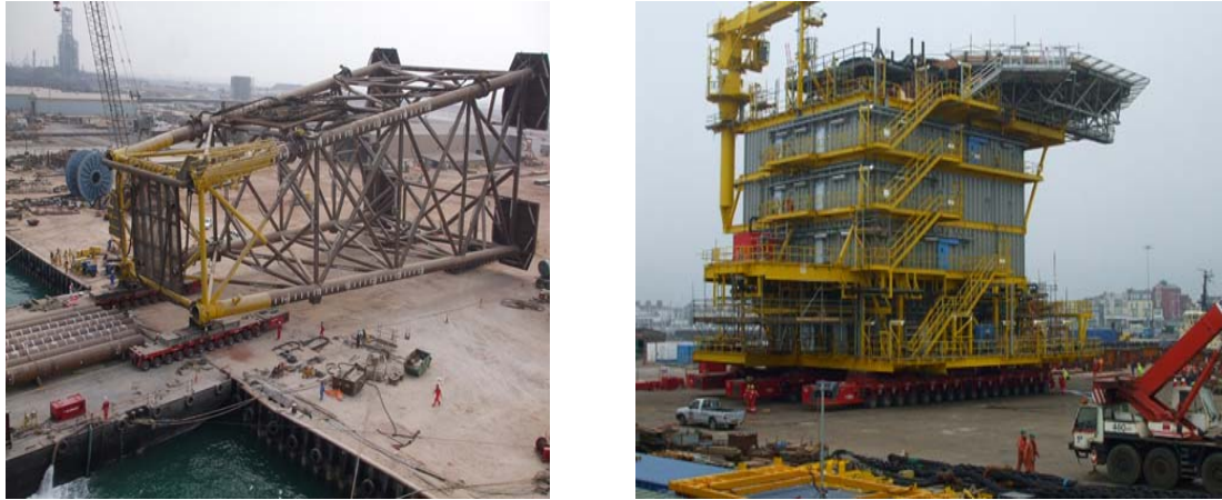
Figure 6 Loadout process (Alyafei and Maerskoil Qatar, 2009)
