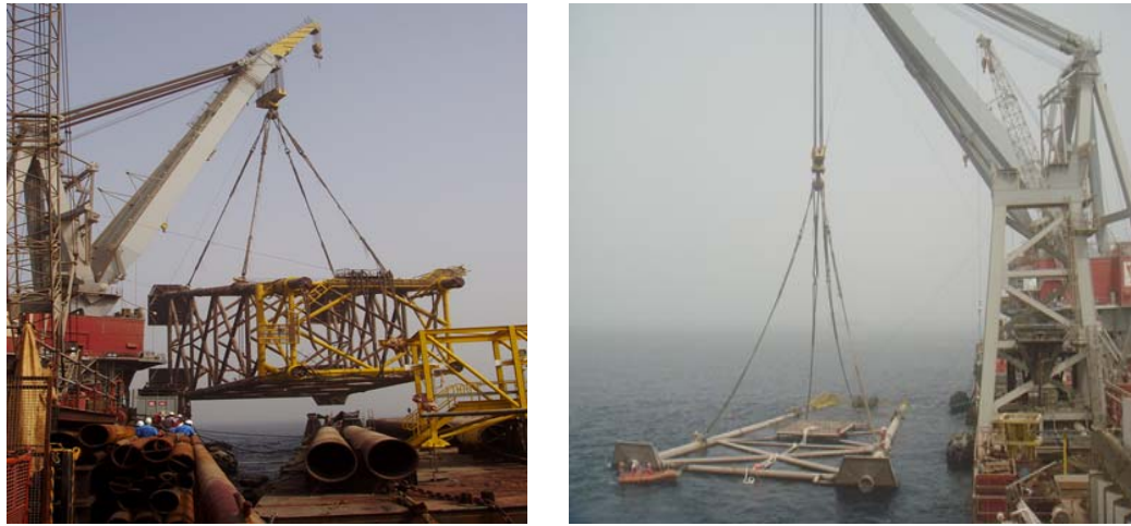
Figure 8 Lifting the jacket and then lower it into the sea (Alyafei and Maerskoil Qatar, 2009)
