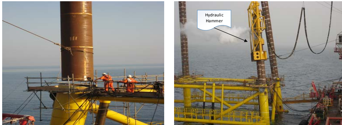
Figure 11 Driving the pile by using hydraulic hammer (Alyafei and Maerskoil Qatar, 2009)
