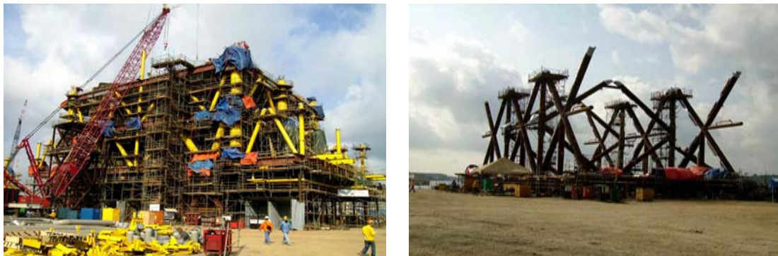
Figure 5 Fabrication yard (Alyafei and Maerskoil Qatar, 2009)
