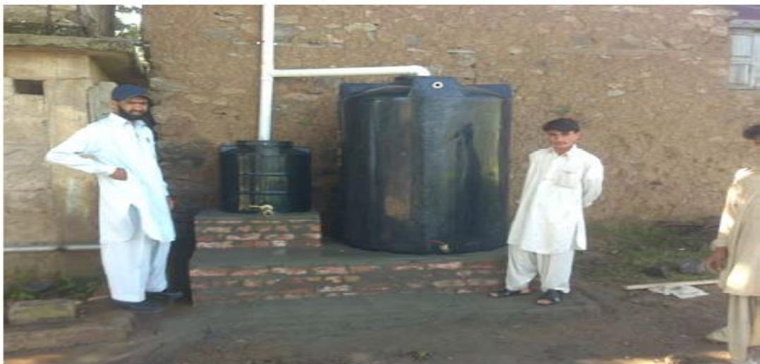
Figure 3. 10 Rooftop RWHS with the addition of first flush diverter
