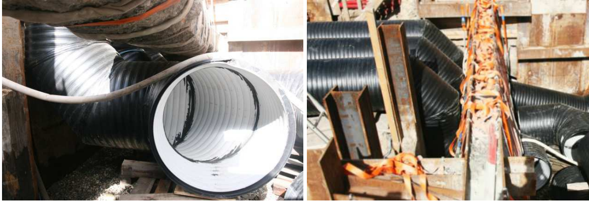
Figure 1. Cloudburst pipes barely able to pass between existing utilities.
