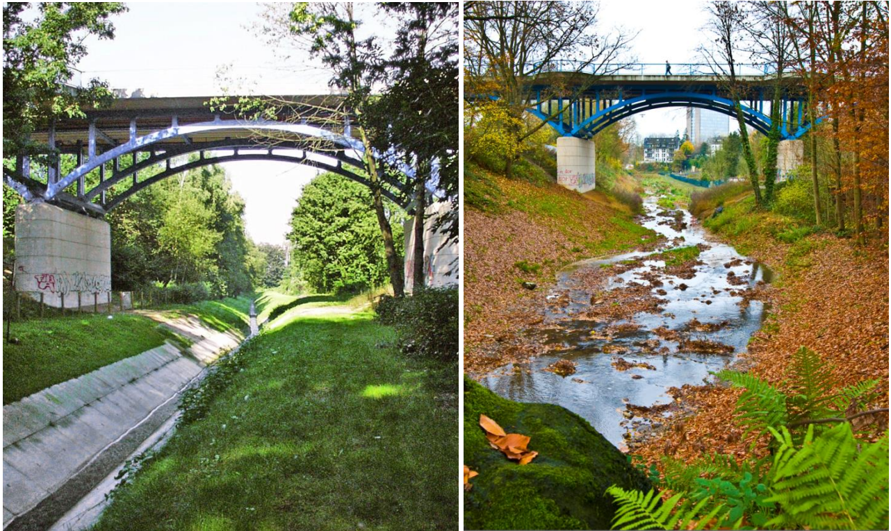
Fig. 1: The Borbecker Mühlenbach as an open wastewater sewer (left) and one year after the ecological improvement (right)
