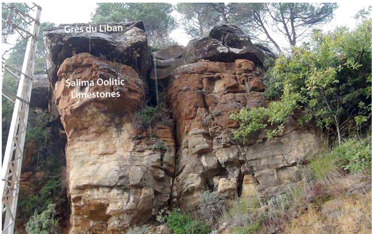
Figure 4: Contact of the "Grès du Liban", here sandstones (above), and the Salima Oolitic Limestones (below). Ain Al Soufsaf ( 33^{\circ}54'13.99''\text{N} , 35^{\circ}44'05.74''\text{E} ), near Mrouj, Matn District.
