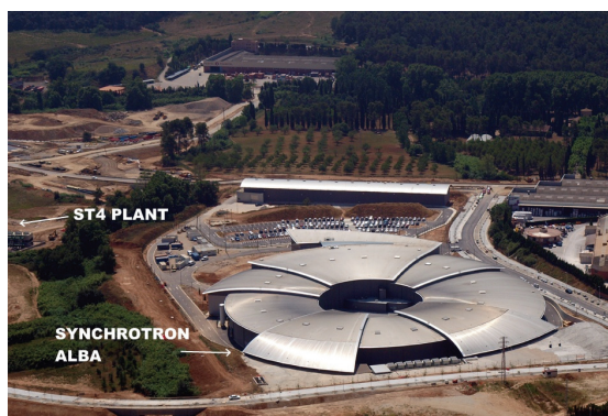
Figure 7.13 Synchrotron ALBA and ST4 plant
