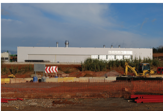
Figure 7.12 General view of the ST4 finished
