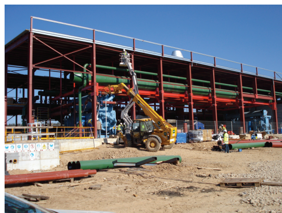
Figure 7.11 ST4 plant during the construction
