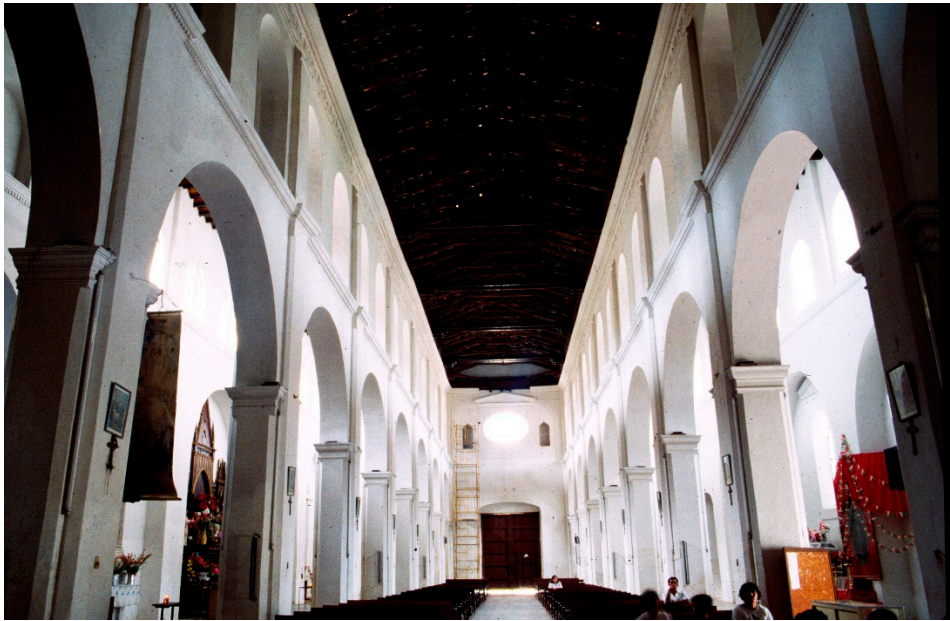
Figure 5. Interior of Santo Domingo church. Chiapa del Corzo. Photo took by author.
